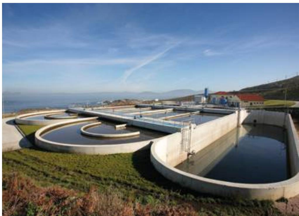
Treatment is of the activated sludge biological type or by prolonged aeration with two carrousel reactors aerated by surface rotors, a prior storm tank and secondary clarifying. Drying by centrifuge.
