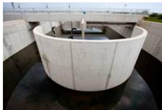
The WWTP is based on an activated sludge system at very low load, that is, with prolonged aeration using a carrousel with two channels. It also has new covered pre-treatment, a new secondary clarifier, deodorising by bio filter as well as new physical and chemical treatment in case the biological treatment is put out of service by an emergency.
