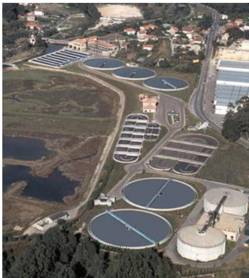
The WWTP is designed for an equivalent population of 400,000, hab. average flow of 1,500 l/s and a peak flow of 3,000 l/s.
