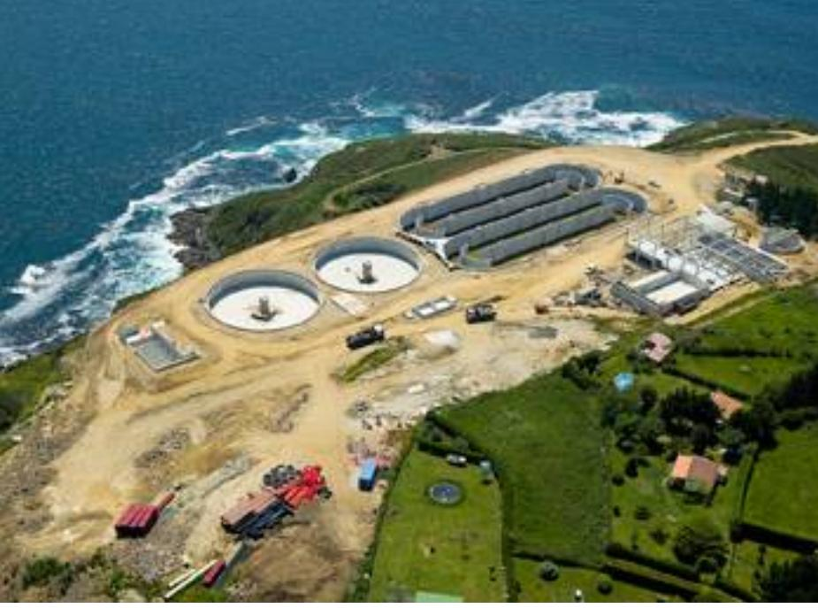
The project consisted of a set of gravity sewers, pumping stations and conduits to lead the sewage from the municipality of Ares, Fene and Mugardos to a single treatment plant in Ares, where it is treated and then discharged to the sea through an outfall. At the same time it was also necessary to build approximately 7 km of power lines to supply the plant with electricity.
