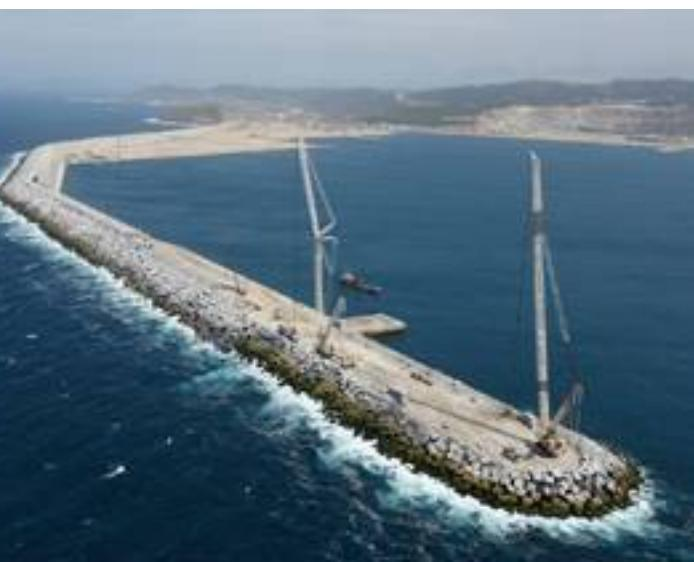
A transverse mole of precast concrete caissons (51.10 x 20.50 m) with a depth varying from 21 to 27 m long. An edge beam 5.35 m deep is located on the caissons to support the outer rail of the crane, the mooring bollards and the fenders. The crane's inner track is 18 m from the outer one on a 1 m beam with a concrete slab 45 cm thick between the two rails.
