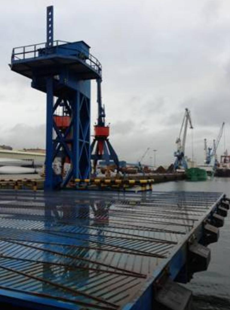
The works under this project are located at the end of the dock, where the North and Fernández Ladreda closing piers meet. There the foundations are at -6 (where Fernández Ladreda pier is grounded) and -10, the latter results from the dredging done to recently build the North pier.
