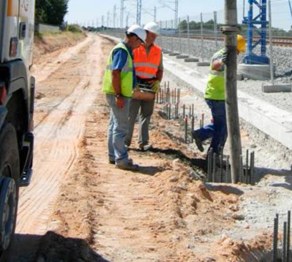
The works consist of installing a number of soundproofing screens at various points along the section of the High-Speed platform between Segovia and Valdestillas, where the noise levels have been found to exceed the permissible fixed limits.
