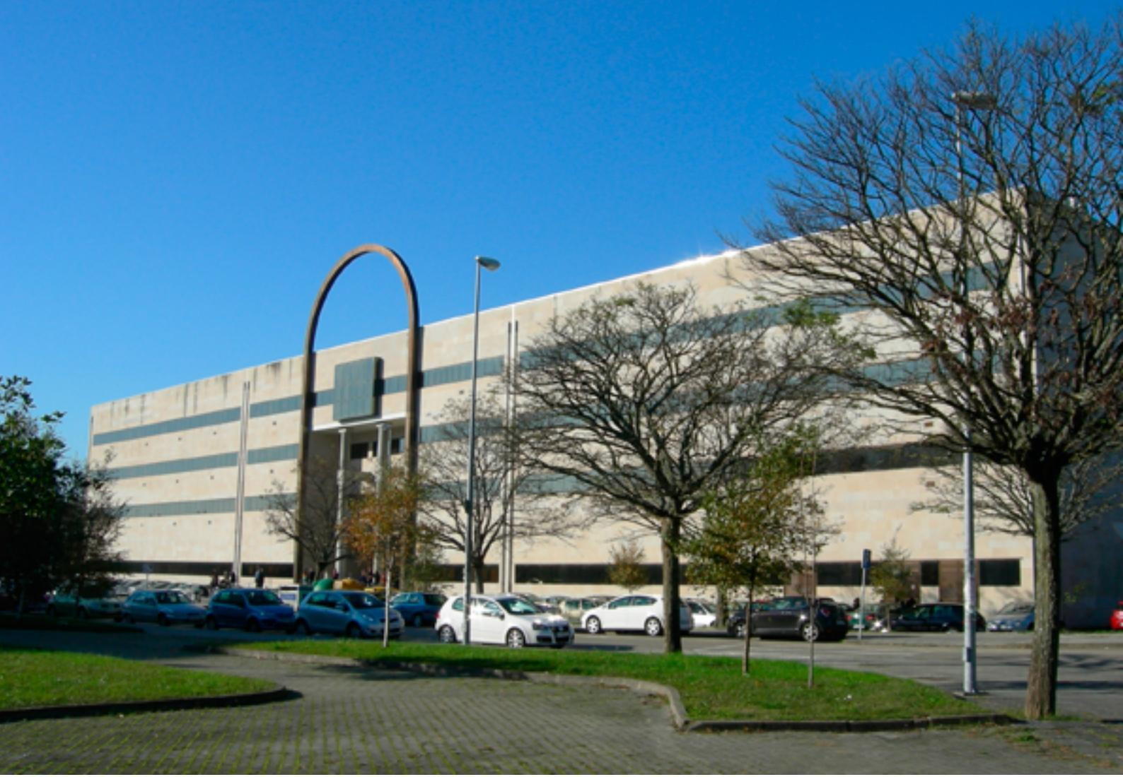
The cladding of the façade comprises a 5 cm thick granite veneer,  $\frac{1}{2}$  foot double hollow brick, air chamber, insulation and a double hollow brick partition. The exterior finish material is aluminium (structural system). For interior partitions, facing brick masonry was used.
