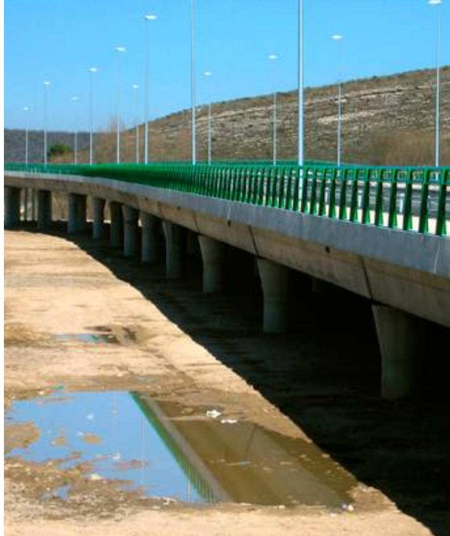
The total deck width, of 21.50 m, consists of a 13 m carriageway, two 2.50 m walkways, and a 2.50 m bicycle lane which is separated from the carriageway by a 1 m walkway. Finally, to ensure the continuity of services for the future industrial estate, water supply and drainage pipelines and electric power lines were installed, both in trenches, directly underneath the deck, and overhead, suspended from the bridge where it crosses the river Ebro.
