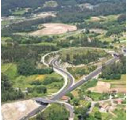
7 flyovers have been constructed with a total length of 206 m. Six of these are portal frames with pillars in a V-shape, and one of them crosses over a span of 24 m using double-T beams, supported on floating abutments on breakwaters. Four underpasses have also been constructed, with a total length of 85 m. They are reinforced concrete portal frames.
