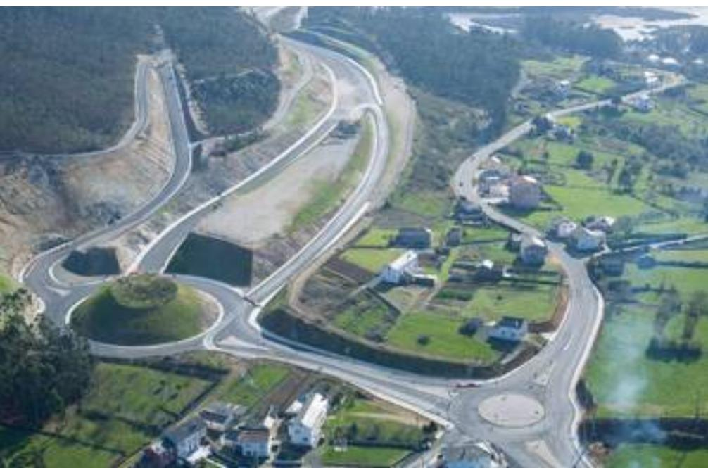
along a hillside in the town of Ortigueira, with cuts of up to 48 m and fills of 35 m. It has three diamond junctions at different levels, four flyovers and two underpasses, a rest area and two viaducts; one of 105 m to cross over the Ortigueira Norte roundabout and the other of 330 m to cross over the river Baleo. The carriageway section consists of a deck of two
