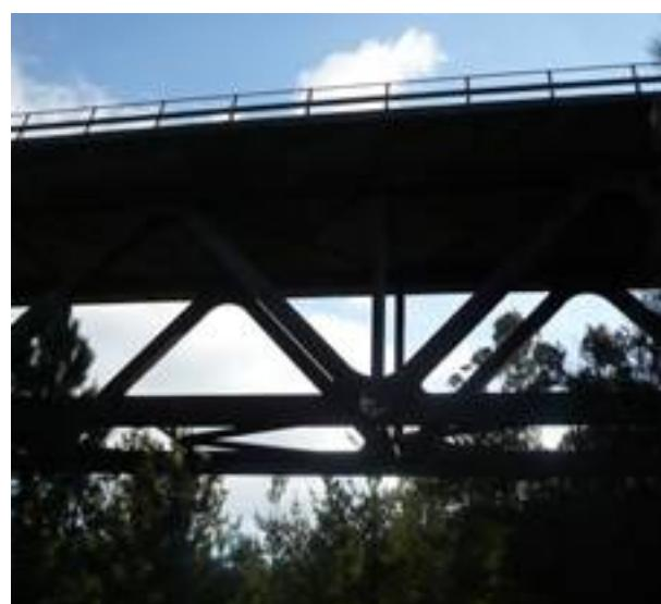
From a technical perspective, the most important feature of this work is the viaduct, with a composite structure of concrete and steel which crosses the river Deva, with three spans of 84 + 120 + 84 m and approximately 65 m above the river.
