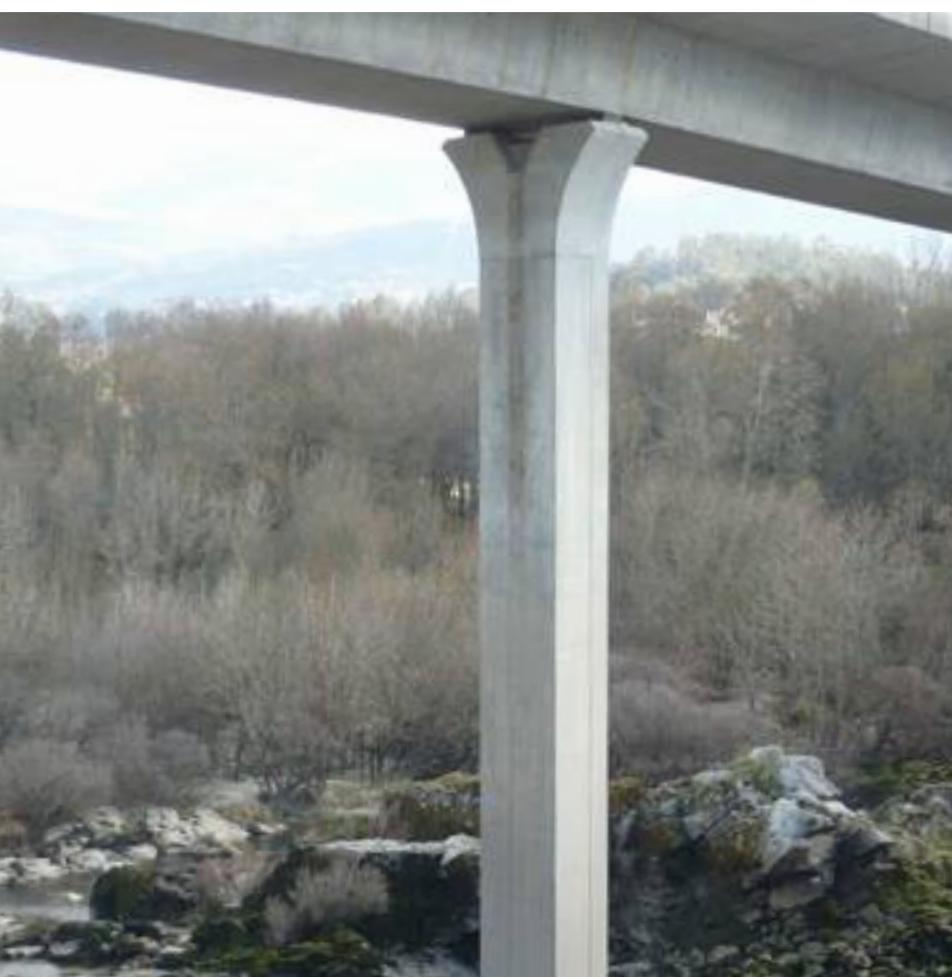
This consisted of constructing the first fixed crossing between two countries in the European Union to be entirely developed by an autonomous community. The works consisted of the construction of a bridge over the river Miño, with a total length of 252 m and approximately 35 m above the waterway, and an access road from the PO-400 road to the bridge. Additionally, in Portugal, the bridge was connected to the road network via a new road which is 600 m long.
