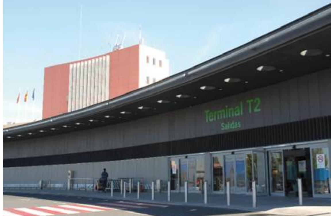
of the new facade was carried out by installing this metallic structure which performs the function of cladding the facade and from which the shelter, with a projection of 4 m, is supported. The entire metallic structure was clad by a ventilated façade with a prefabricated element which conforms to the curvature of the building. Some sunshades have been installed on the façade at a specific height and angle to enable light to enter the terminal.
