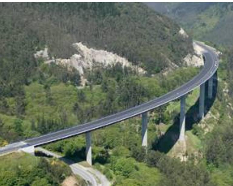
Selecting a composite structure made it possible to widen the section from 11.50 m to 23 m, simply by putting metal struts in place and concreting over the rest of the slab.
