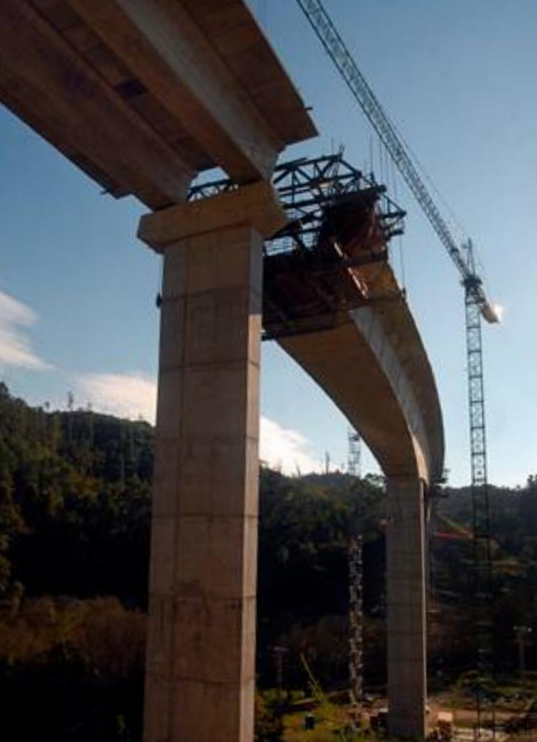
The Caldas de Reis bypass crosses over the valley of the river Umia at a height of 40 m, and a viaduct has been designed which is 456 m long, distributed over 7 spans, with the following layout: 4 x 39 – 75 – 150 – 75 m.
