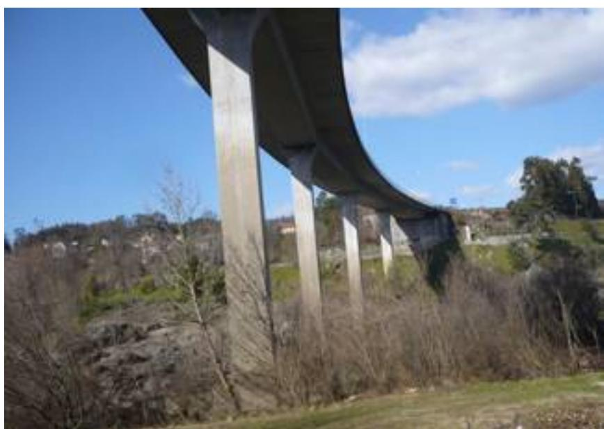
Given the special topography and the heritage protection in force in this location, the presence of people fishing lamprey in this area of the river, the method chosen to construct this bridge was almost exclusively prefabrication. Therefore, both the girders and the pillars, with a maximum height of 28.00 m, were prefabricated and transported to the location of the bridge, where they were assembled using cranes with a maximum capacity of 650 t.
