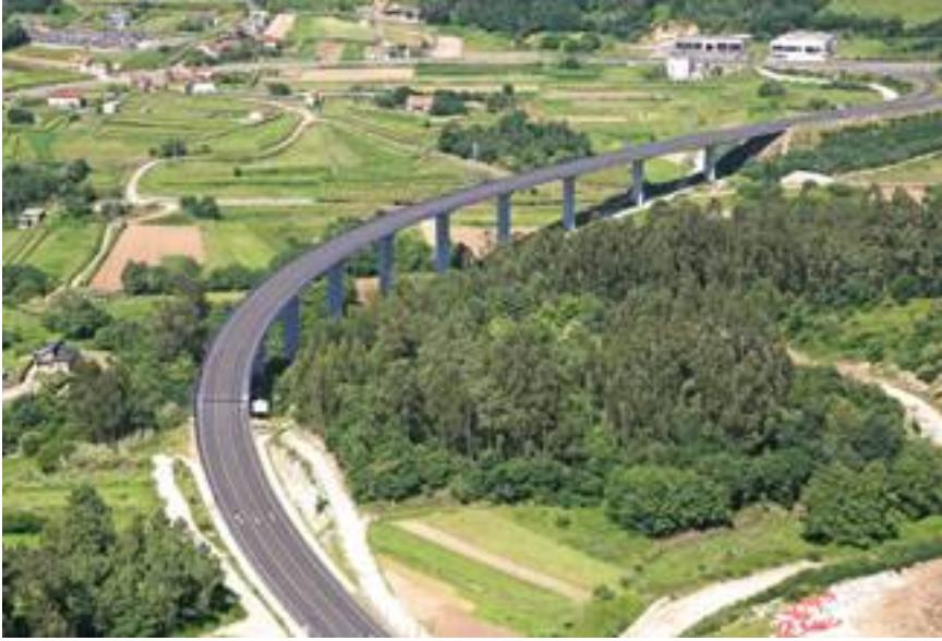
The deck of the viaduct consists of a post-tensioned concrete girder box with the following sequence of arch spans: 46.75 – 9 x 55.00 – 46.75 m.
