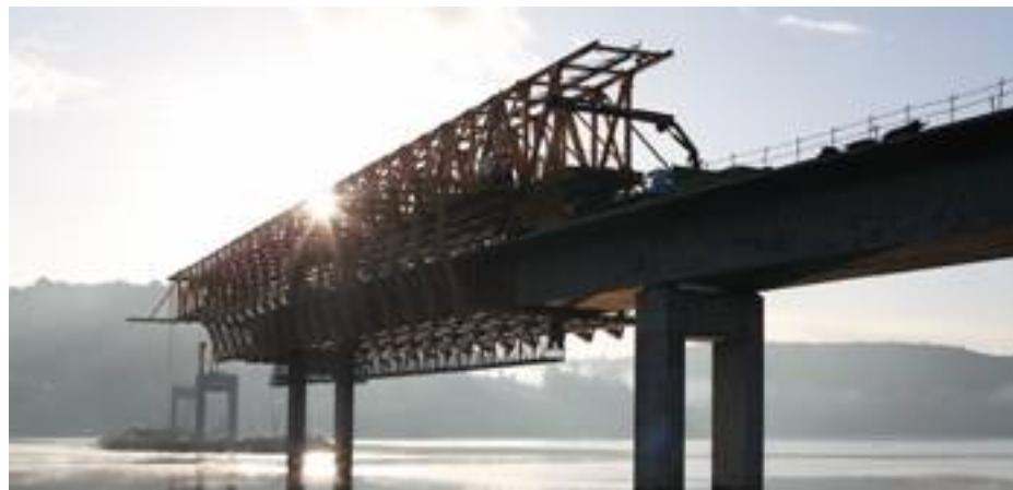
Although this is a simple structure with pillars which are low in height, the main feature of this bridge was the span of its arches, which was 70 m, making this the first bridge to be built using movable formwork with such a high span length.
