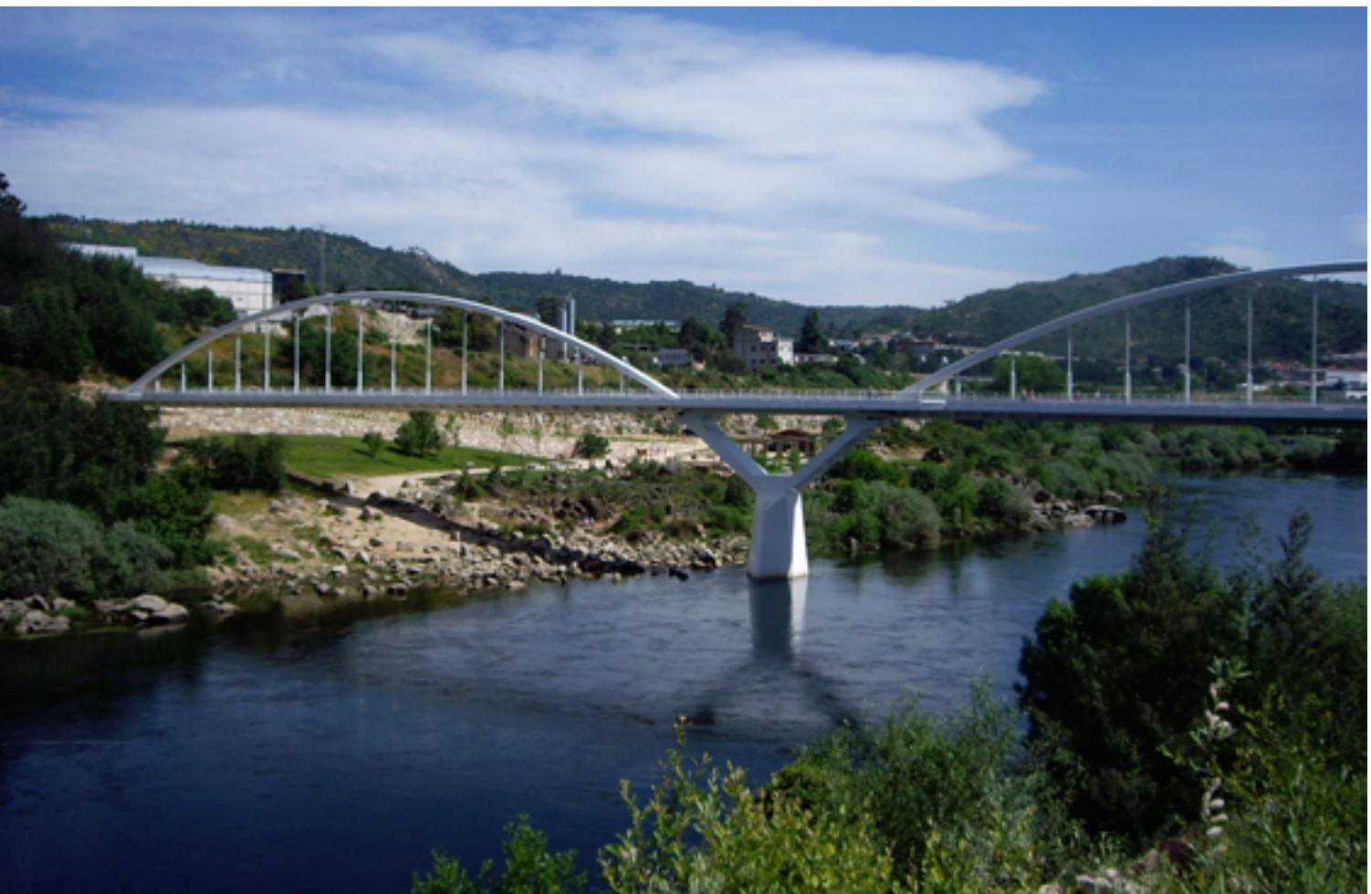
The project involved two actions. Firstly, the riverside was conditioned by protecting the banks against erosion with riprap and a “green blanket” in which green areas and paths were provided, the existing ones conditioned and equipped with lighting and automatic irrigation provided for the gardens.
