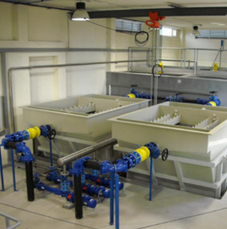
After the exit from the filters, post-chlorination takes place using sodium hypochlorite.
