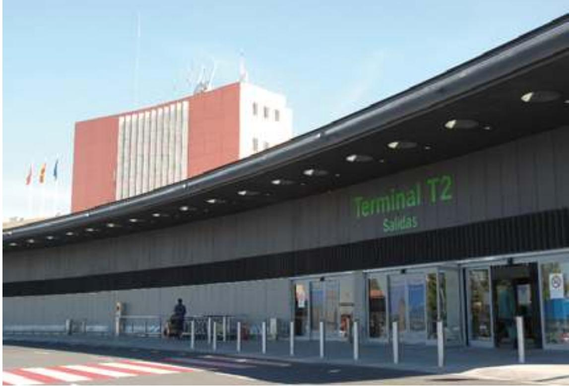
of the new facade was carried out by installing this metallic structure which performs the function of cladding the facade and from which the shelter, with a projection of 4 m, is supported. The entire metallic structure was clad by a ventilated façade with a prefabricated element which conforms to the curvature of the building. Some sunshades have been installed on the façade at a specific height and angle to enable light to enter the terminal.
