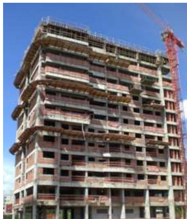
The foundations used are mixed, with metal driven piles and on site piles. The structure is concrete and the exterior finish materials combine tiles with painted plaster and aluminium cladding.
