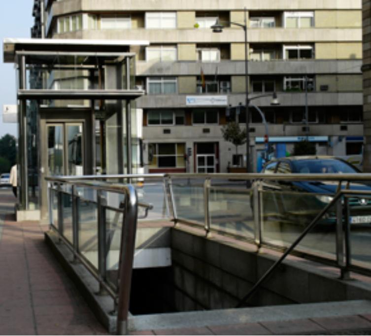
The interior width of the construction is 15 m, divided into two sets of 5 m parking spaces, a central aisle which is also 5 m, with the fully completed construction being 650 m. The floor area is approximately 10,500 m<sup>2</sup>, with a resulting 496 parking spaces.
